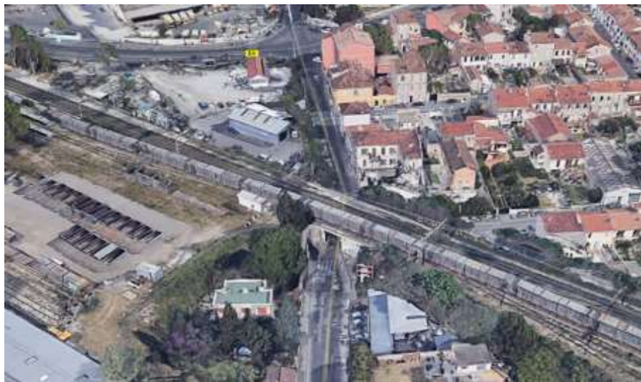
Figure 69 : Pont rail de l'avenue Ibrahim Ali (Google Earth, 2021)
